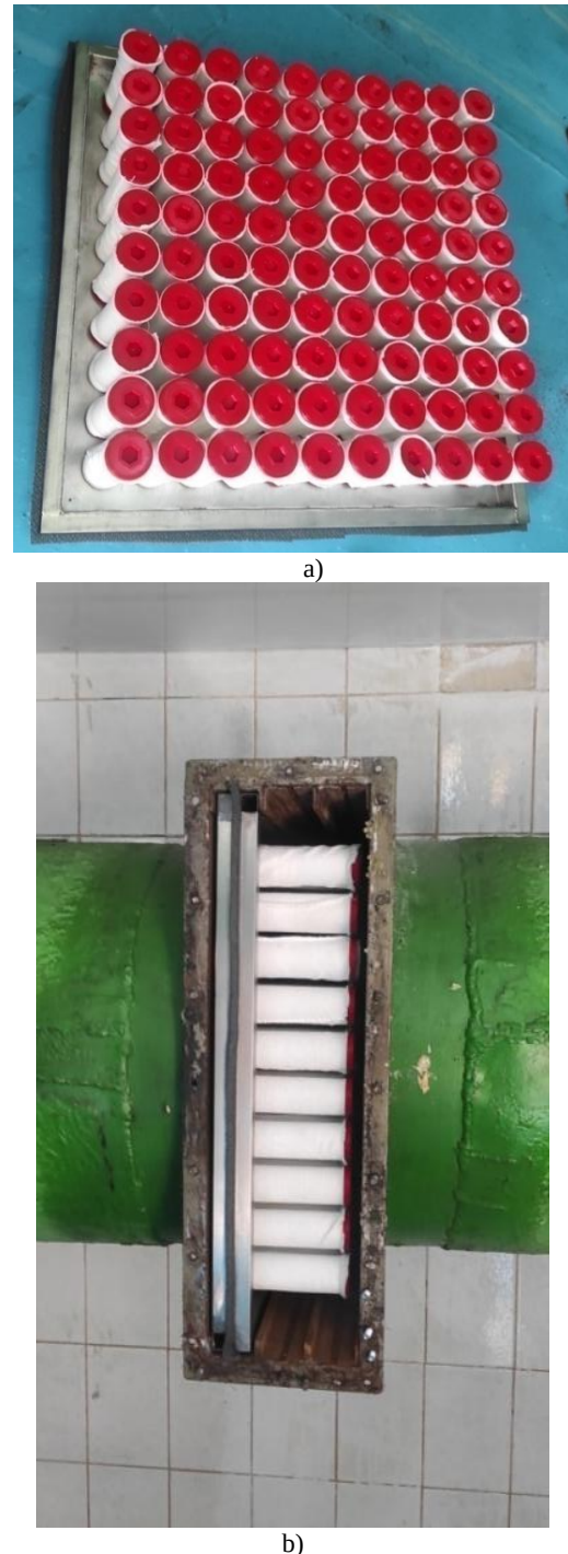
Fig. 3. Air cleaning filter (a) and mounted in the air supply system (b) external view. (Photographer: I. Charniak)
